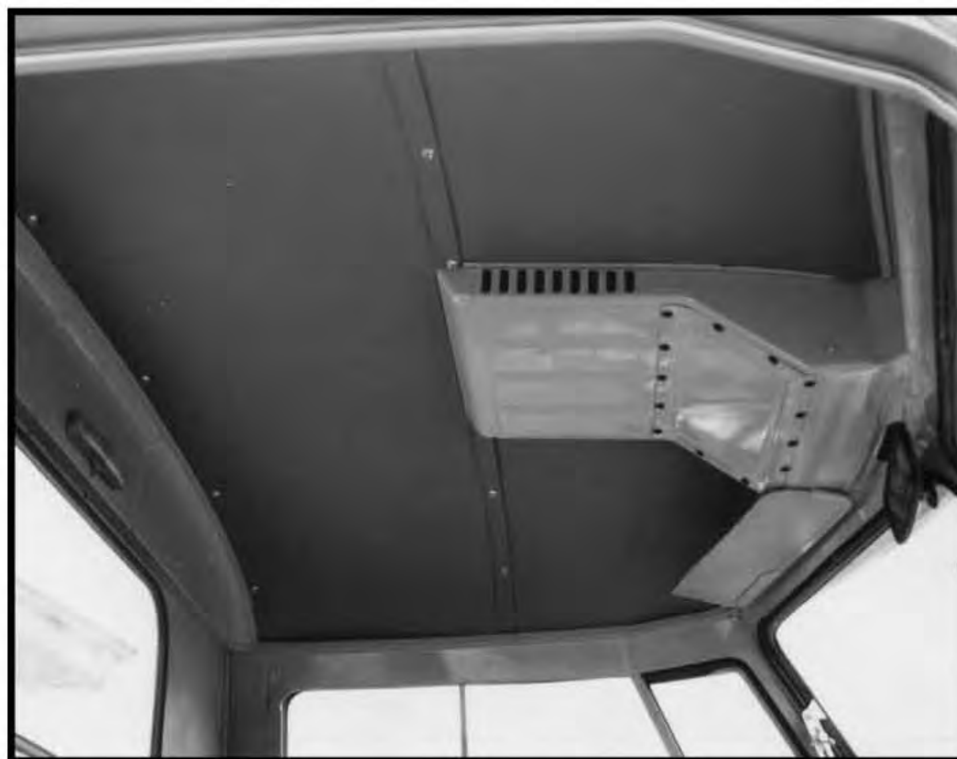
New Headliner Installation
